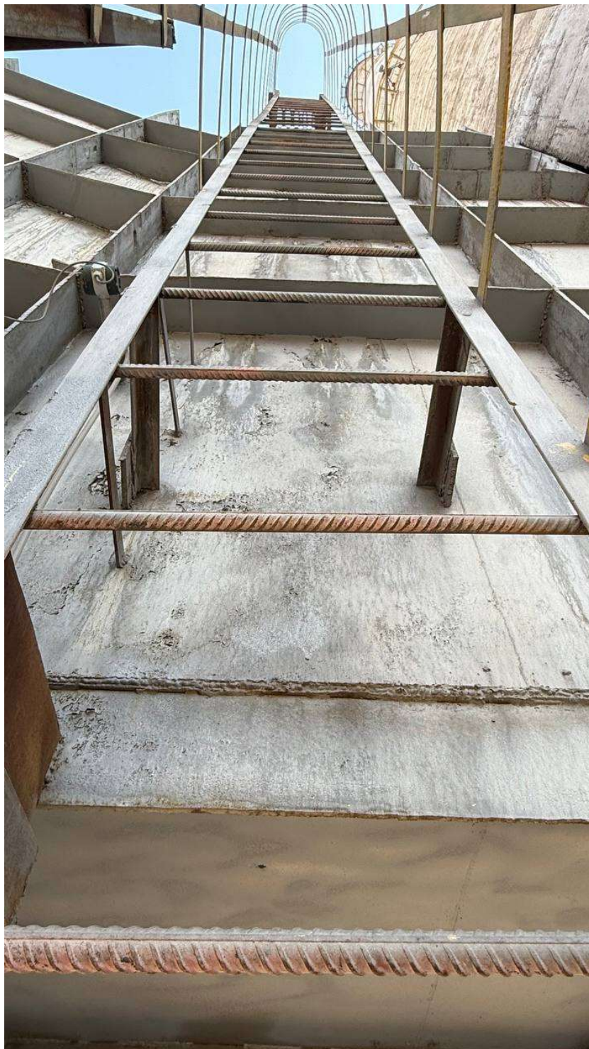
26-rasm.. Gazoxod inshootining texnik xizmat ko‘rsatish zinapoyasi (vertikal narvon) ko‘rinishi
