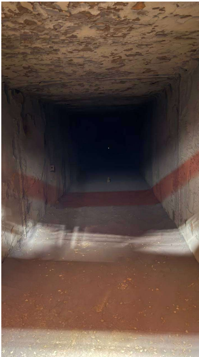
45-rasm. Gazoxod trubasining ichki qismi holati (vizual ko‘rik natijasi)
