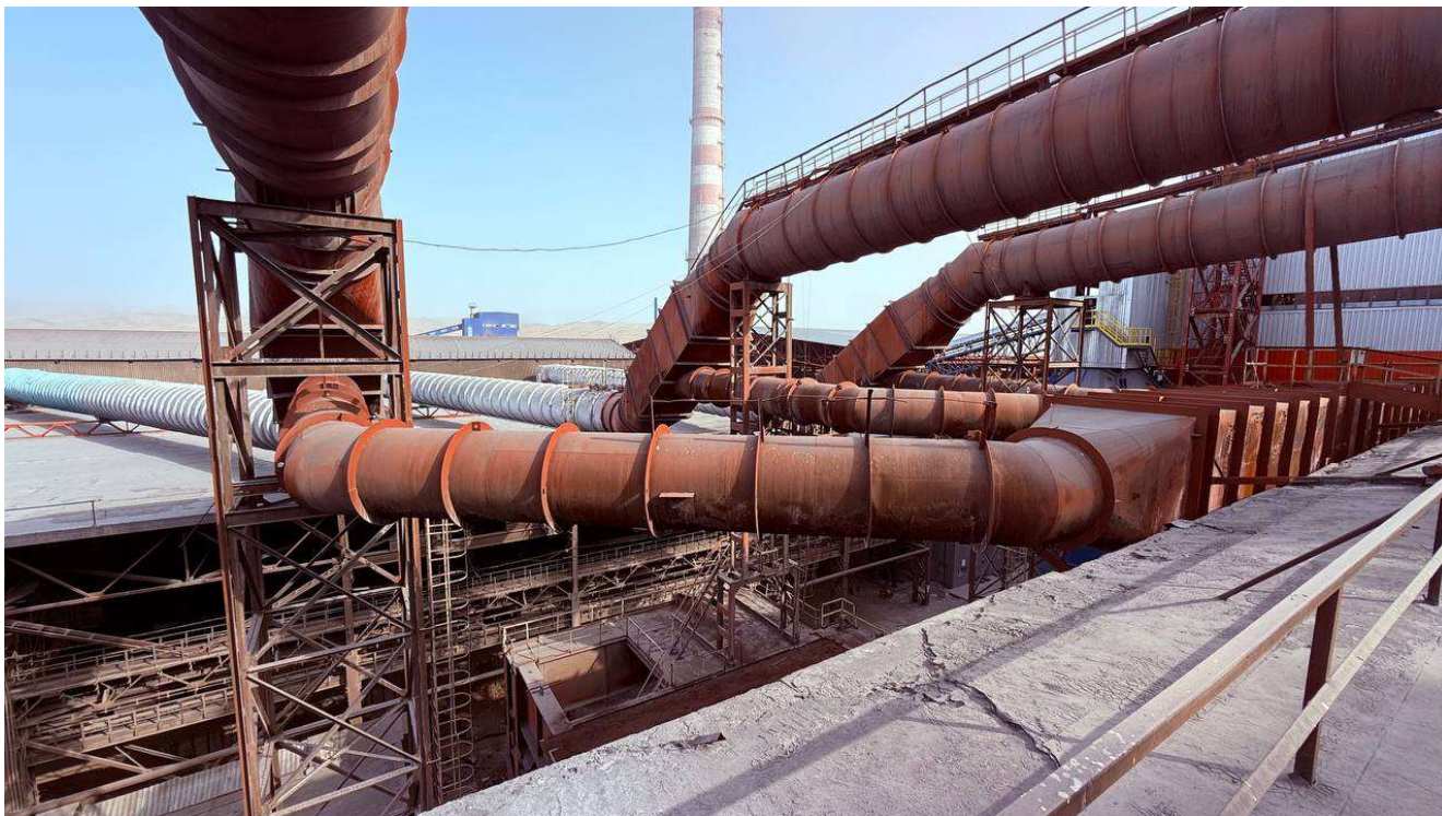
2-rasm. Elektrda po‘lat eritish bo‘limining gaz tozalash yo‘li (gazoxod) inshootining tashqi ko‘rinishi.
