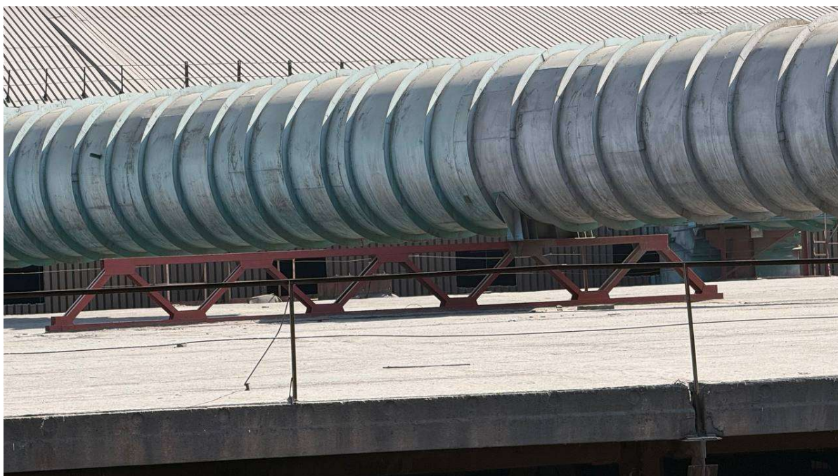
54-rasm. Gazoxod trubasining tom ustidagi qismi (tashqi ko'rinishi)
